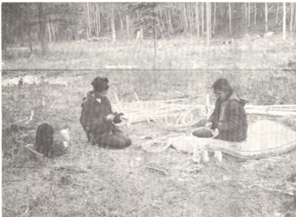
Peeling spruce roots to use in log building construction are these women of Mentasta, workers in a project to create an authentic Indian village for visitors and travellers along the Glennallen highway. The peeled roots tie logs together; traditional log buildings have no nails.
