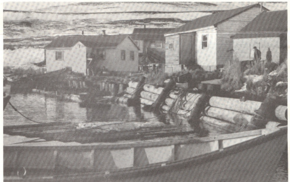
New protection against high water will be provided these Akhiok homes by the new log bulkhead shown here. The project was one of a number of village improvements funded by Operation Mainstream and carried out by Akhiok residents.
