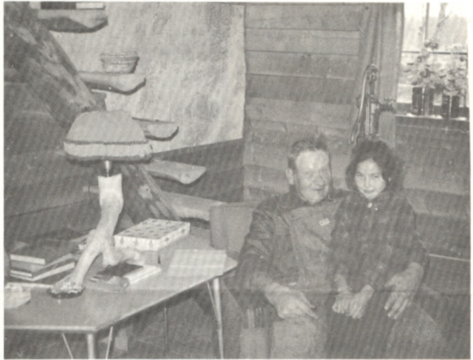
Walter Sellens, BIA supervisor for the housing project in Lower Kalskag, is shown here inside one of the new houses he finished himself with his young friend, Miss Dora, niece of the local supervisor, Sinka Williams. Local residents in the village completed 17 log houses last month. The homes were built during the process of moving the village back from the Kuskokwim River. The project was sponsored and funded by BIA. Operation Mainstream sponsored by RurALCAP, assisted by providing $17,000 for training men in construction of homes.
