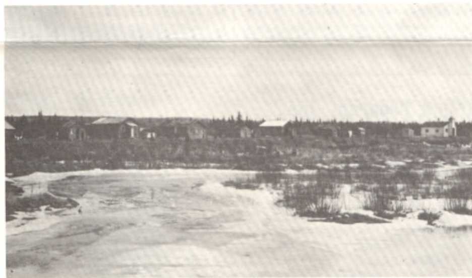
The village of Alakanuk, located on the Bering Sea, is slated to build a community hall for village activities. Meetings are presently held in an abandoned church building not belonging to the village, and the villagers make only necessary minor maintenance repairs.
