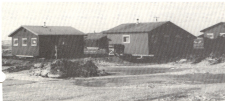
The new houses have been moved from the factory site to the other side of Brown Slough in Bethel. The houses shown above are in the "cluster" effect planned for the housing development.
